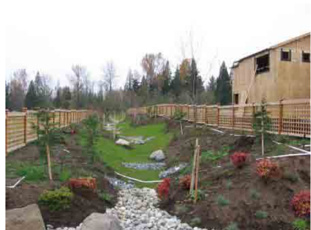
LID swale water is retained on-site.
