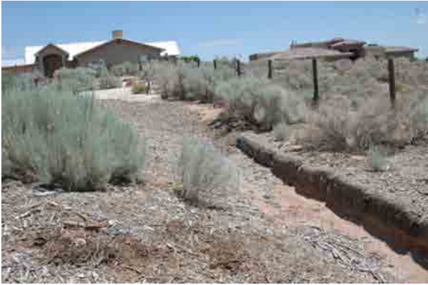
Straw bales, wood mulch and undulating the land allows water to slowly enter this water collection area to protect downstream properties from increased flow rates.
