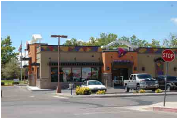
Screen roof-mounted mechanical equipment from view with the use of parapet walls.
