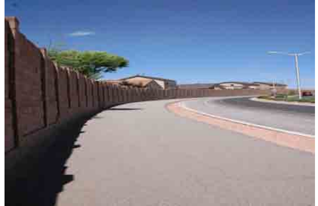
Landscaping with trees shall be located along both sides of a sidewalk and walls greater than eight feet in height shall be stepped with a five-foot horizontal offset with landscaping in the offset.
