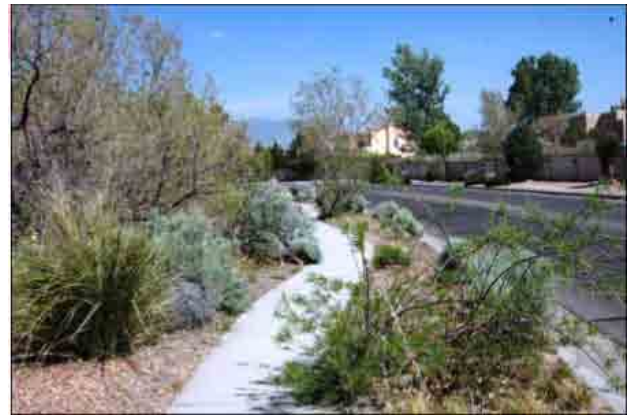
Overgrown landscaping inhibits sidewalk use and cactus should not be located within three feet of a sidewalk.
